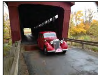
Parker Bridge in Upper Sandusky (built in 1878, burnt in 1991, renovated in 1992 - Howe Through Truss - 182 feet long)
