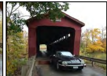
Parker Bridge in Upper Sandusky (built in 1878, burnt in 1991, renovated in 1992 - Howe Through Truss - 182 feet long)
