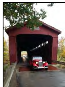
Mintueman Bridge in Clyde (built in 1988 - Stringer Truss - 51 feet long)
