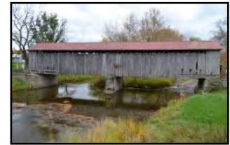
Mull Bridge in Fremont (built in 1851, closed to traffic in 1962 - Town Lattice Truss - 100 feet long)
