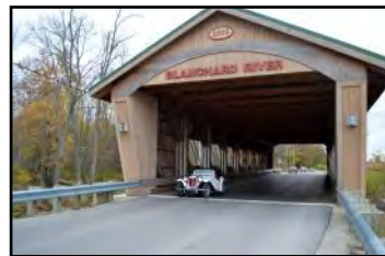
Blanchard River Bridge in Findlay (built in 2009 - Pratt Through Truss - 125 feet long)
