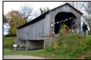
Mull Bridge in Fremont (built in 1851, closed to traffic in 1962 - Town Lattice Truss - 100 feet long)
